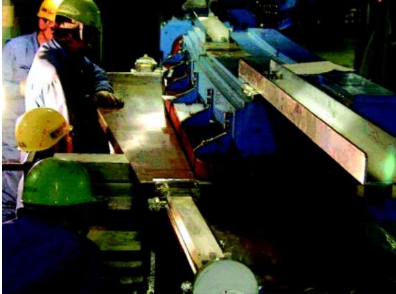
Figure 1. Installation of a vacuum duct for a bending section.
